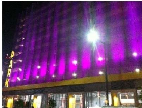
*ACTUAL PICTURE OF PARKING GARAGE*
