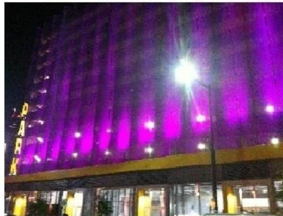
*ACTUAL PICTURE OF PARKING GARAGE*
